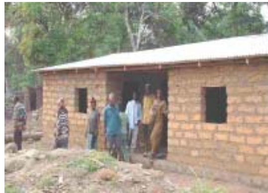
Newly constructed building in Kono District
